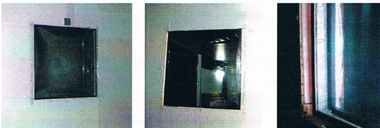
Figure 3. Photos of the installation. Left: view from outdoor side; middle: view from indoor side; right: zoom-in view of the gap between specimen and DGU (the specimen is on the left)
